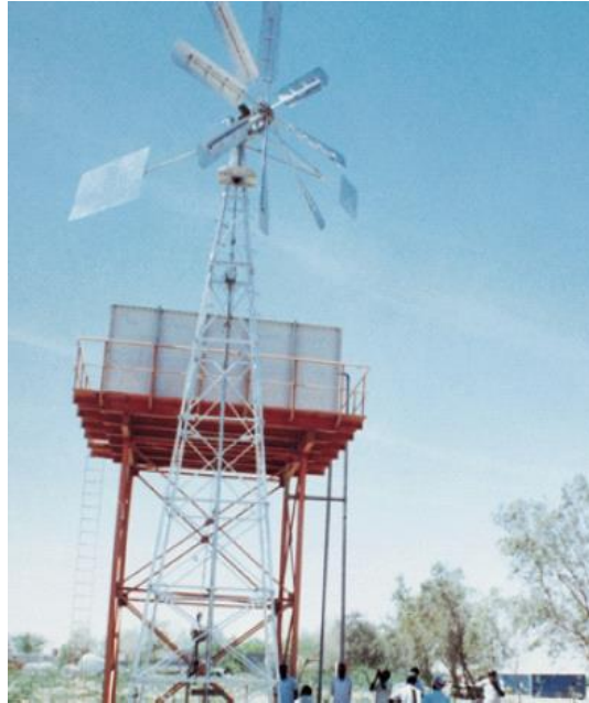
Figure 5. Locally-manufactured wind pump installed at kilo 8 site.
