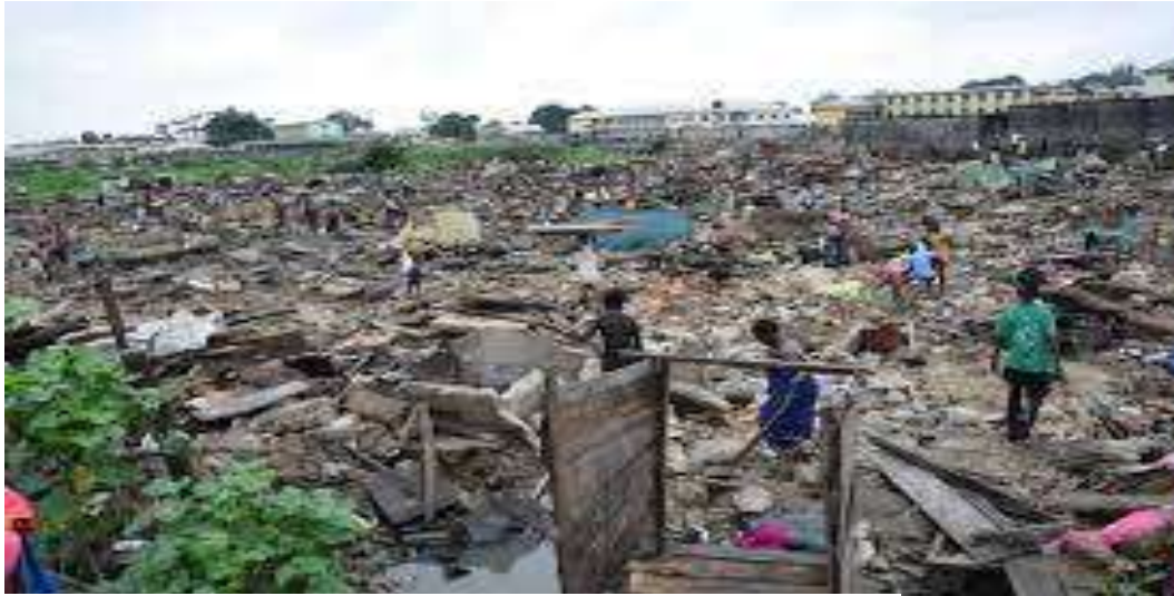
Figure 3: Picture of demolition of Waterfront slums in Port Harcourt Source: www.google.com , 2022
