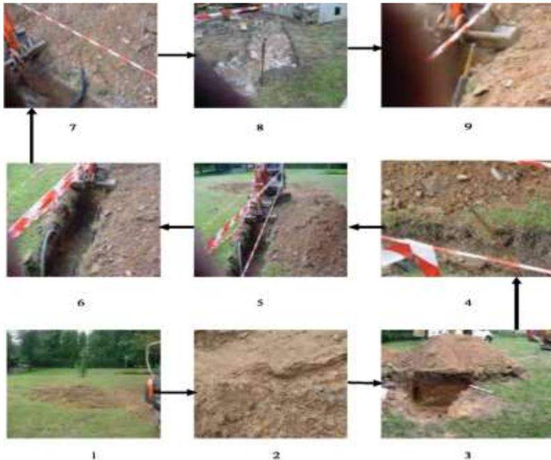
Figure 3. Drilling (1-2) digging of the pit (3), connection of the manifolds (4), grouting, preparation of the coils (5-6) and the source loop, which consists of two earth loops: one for vapour and one for liquid (7-9).
