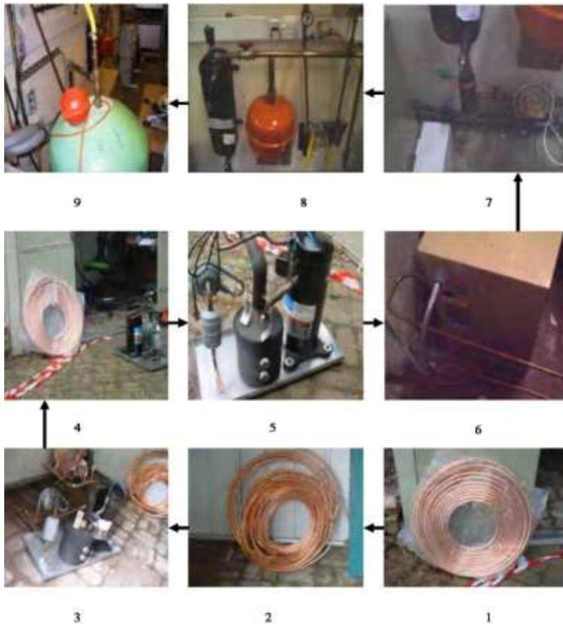
**Figure 4. Preparation of coils (1-2), installation of heat pump (3-6) and connection of water supply system (water pump, flow meter, expansion valve and the boiler) (7-9).**
