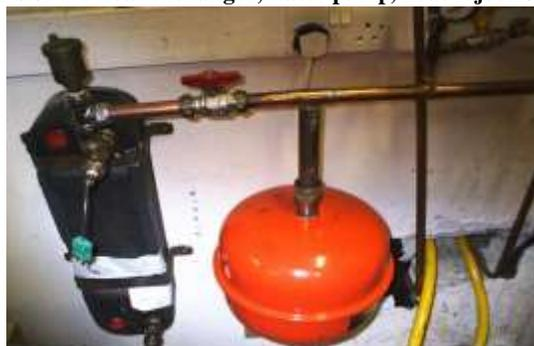
Figure 16. The connections of the heat exchanger and expansion valve.
