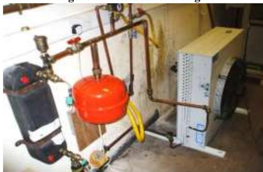
Figure 15. The connections of the heat exchanger, water pump, heat rejection fan and expansion valve.
